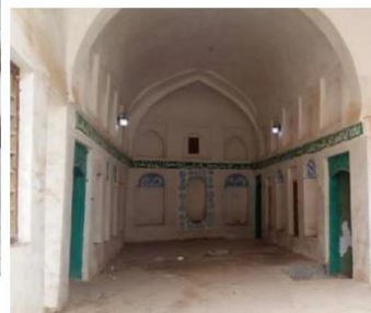
f. Iwan: the roofed part of the yard.
