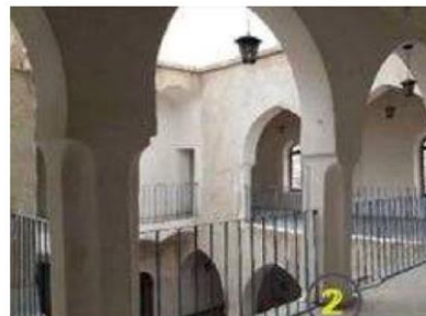
d. Most windows open to the inside.
