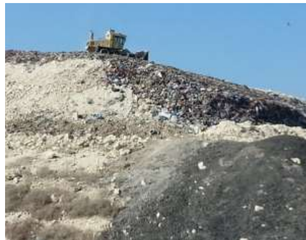
Figure 9 A photo showing the vertical expansion for the landfill
