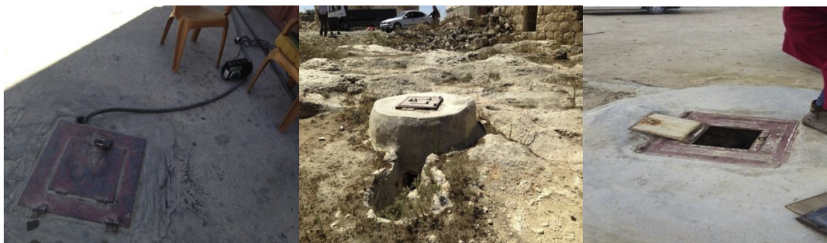
Fig. 3. Representative pictures of the cistern tops.
